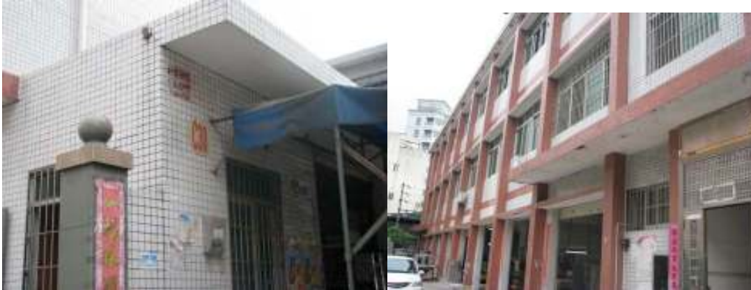
Exterior of Target Factory
