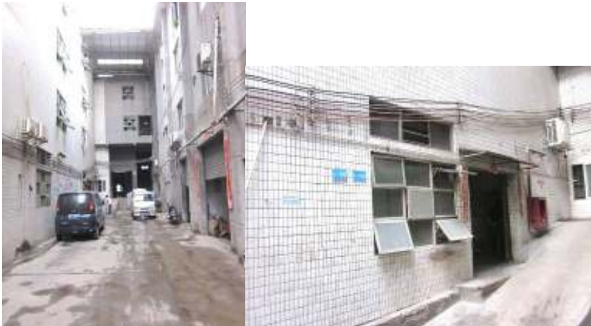
Exterior of Target Factory
